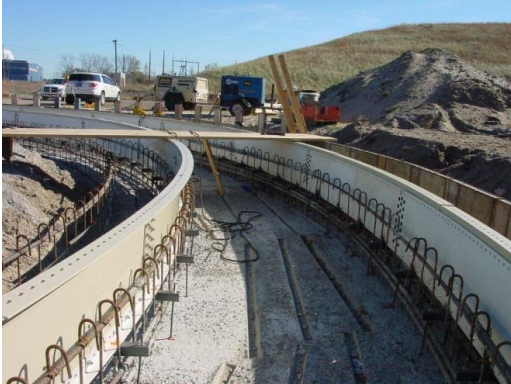
Embedded ring and rebar; ready for concrete
