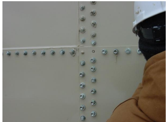
Bolting/Sealant detail
