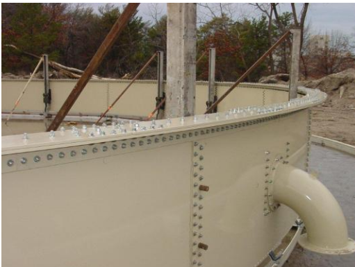
First course, Tank Top. Note overflow elbow.
